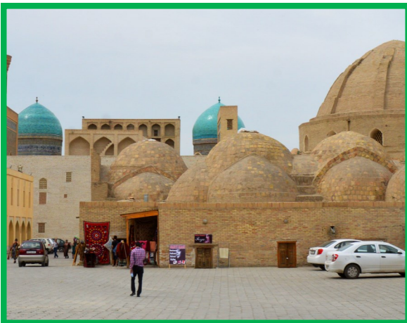
Bukhara: General view
